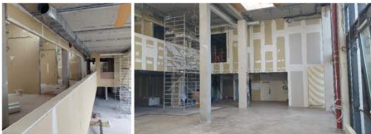
Fig.24: Refurbishment of the ISU library
